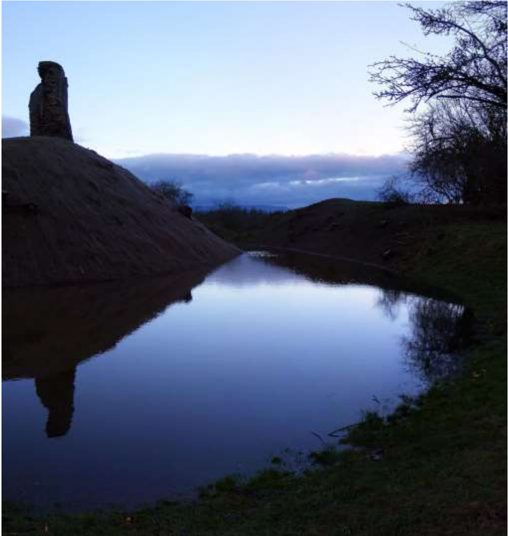
Plate 5.3. Kilpeck Castle following the completion of restoration works
