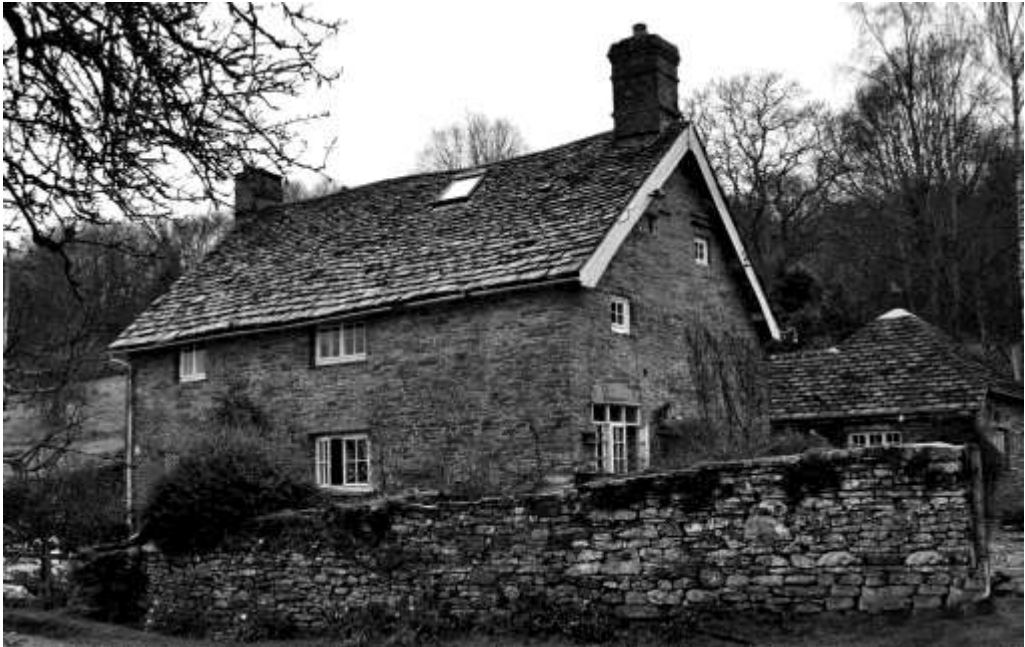
Figure 12. Old House Farm, Bredwardine. North-east elevation
