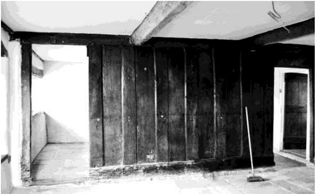
Figure 13. Old House Farm, Bredwardine. The plank and muntin screen, looking south
