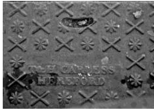
Figure 9. One surviving cellar flap of a pair outside the Chandos Pharmacy, at the junction of St. Ethelbert Street and Cantilupe Street. T. & H. Carless was a firm of ironmongers, subsequently taken over by Harding Bros. The decoration is unusual
