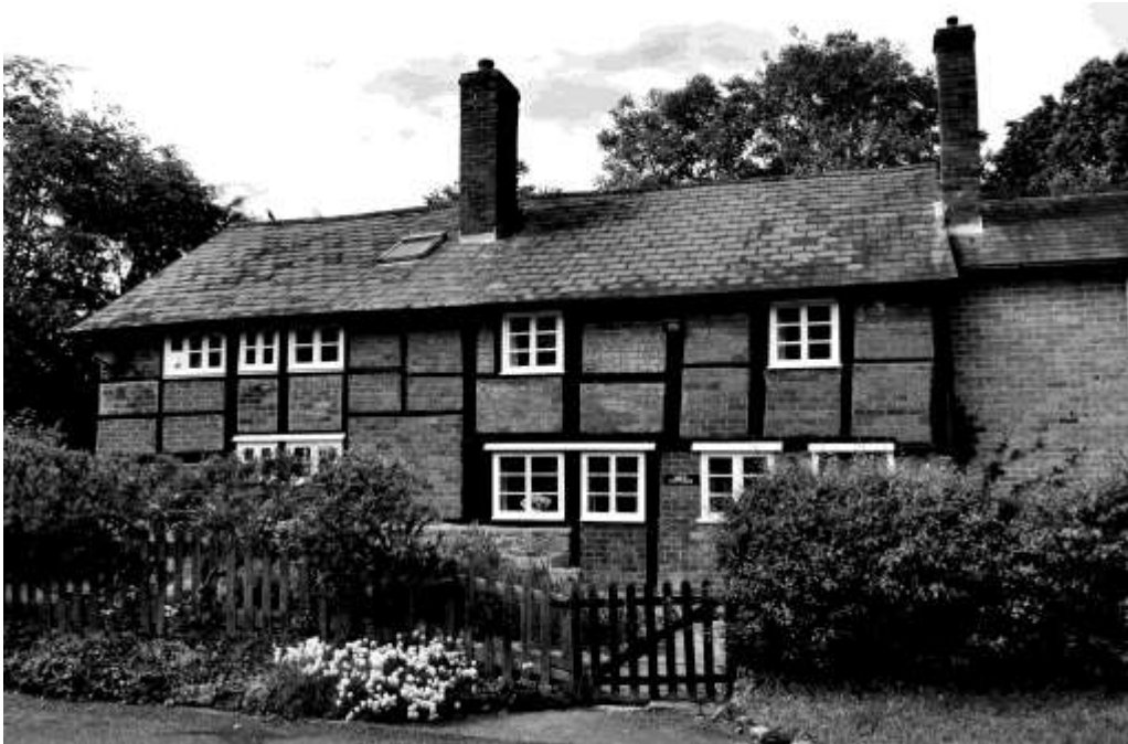
Figure 16. Shop Cottage, Monkland. South-east elevation
