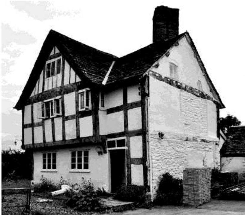
Figure 7. New House Farm, Moccas. The jettied crosswing and single surviving bay of the ceiled hall range
