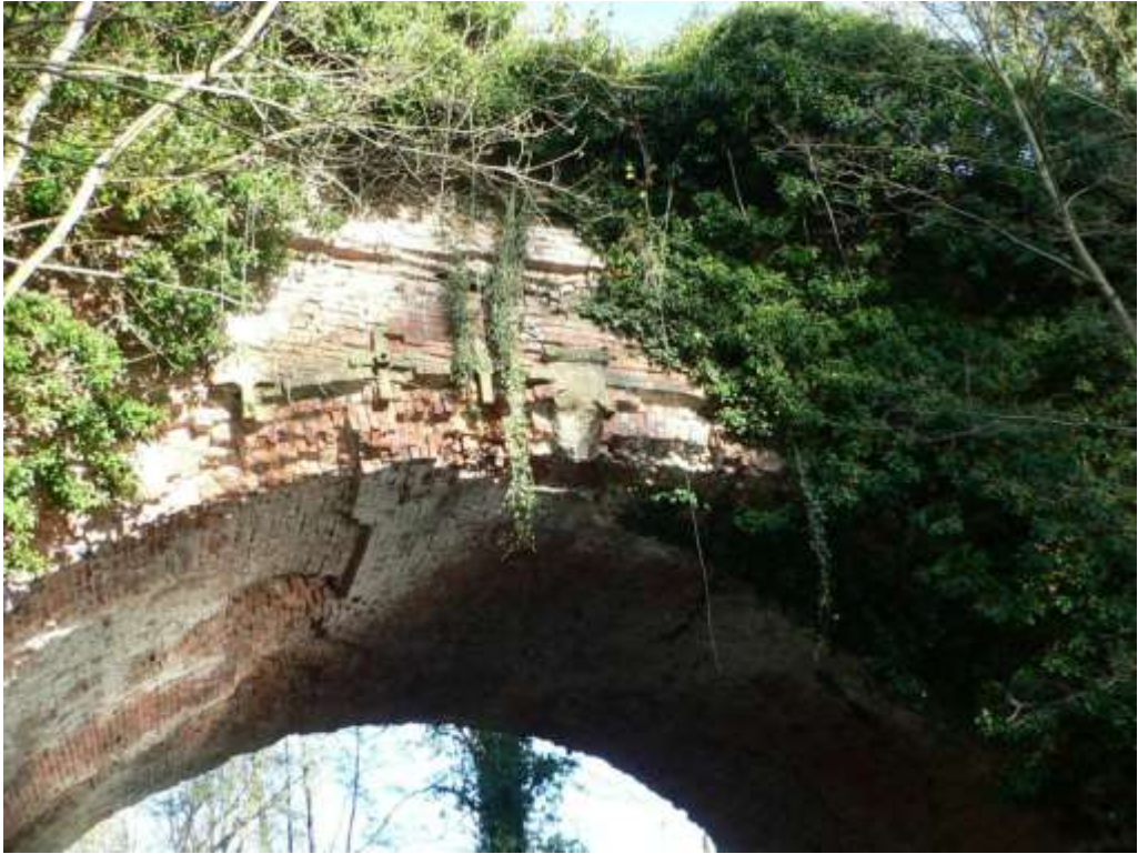
Plate 4.3. The downstream face of the Rea aqueduct, 13 November 2004. (©G. Calderbank)
