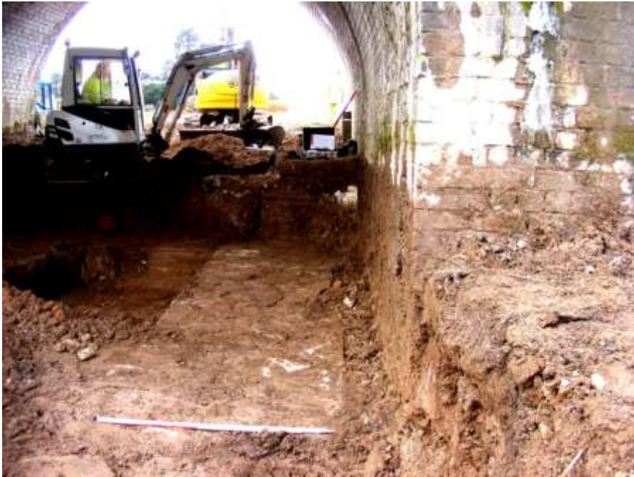
Plate 5.4. Rotherwas. The cutwater for the single-line railway bridge over the Wye
