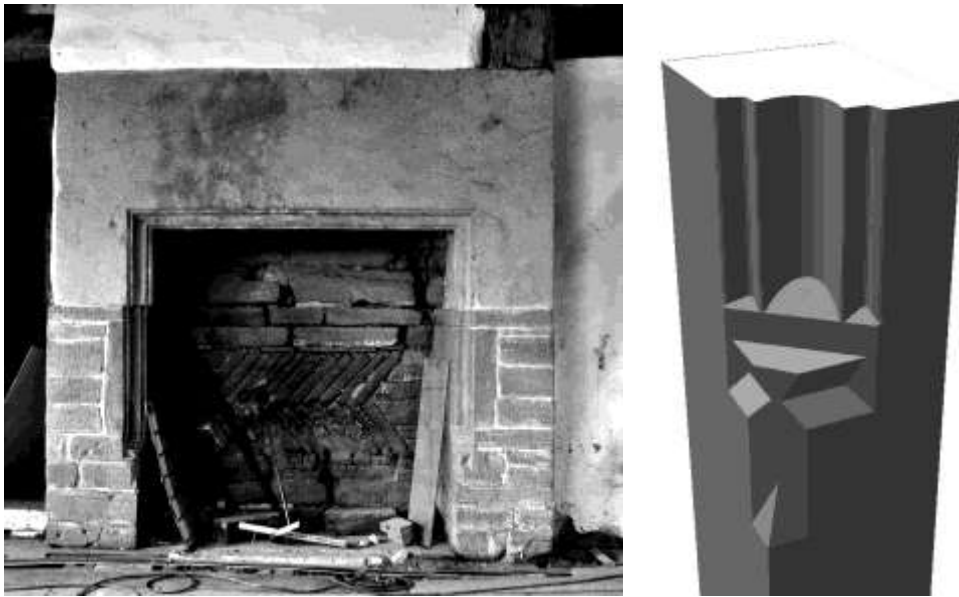
Figure 9. New House Farm, Moccas. The first-floor fireplace in the crosswing Figure 10 (right). Sketch of the moulding profile and elaborate stop on the jambs of the first-floor fireplace in the crosswing
