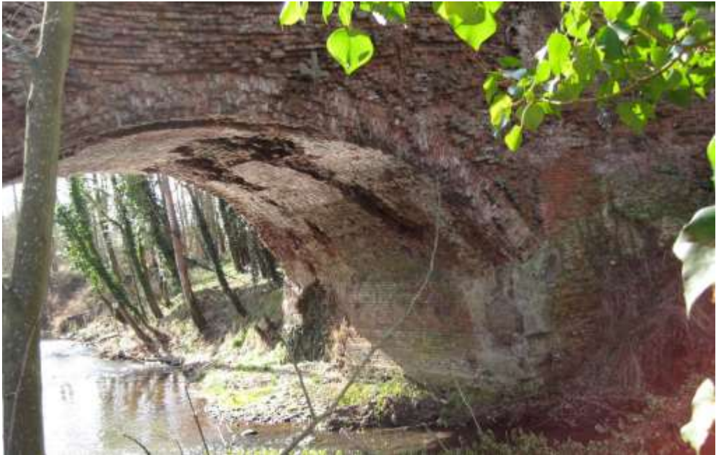
Plate 4.1. The upstream face of the Rea aqueduct before face collapse, 10 March 2012. (©G. Calderbank)
