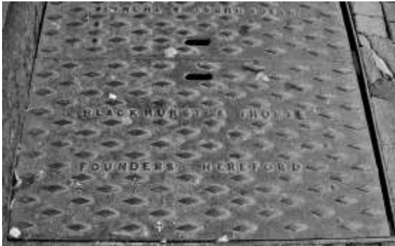
Figure 7. A fine pair of cellar flaps is in the pavement outside The Thai on the Wye in West Street, Hereford, cast by Blackhurst and Thomas, c.1880
