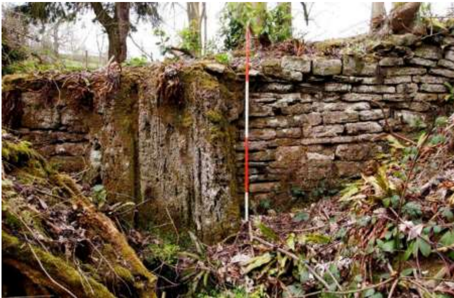
Plate 5.5. Brockhampton. Hyde Dingle. Dam with cascade fossilised in tufa
