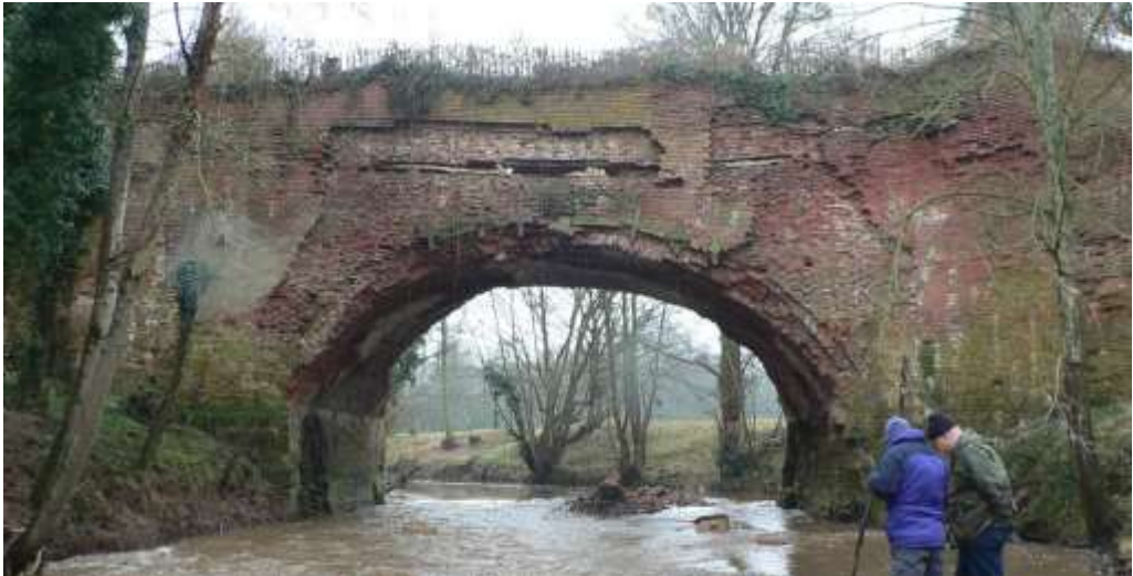
Plate 4.4 . The downstream face of the Rea aqueduct, 10 March 2013. (©G. Calderbank)
