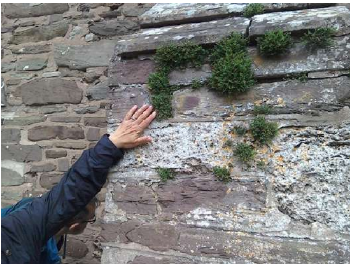
Fig.4 The use of Tufa and local Old Red Sandstone in Bredwardine Church
