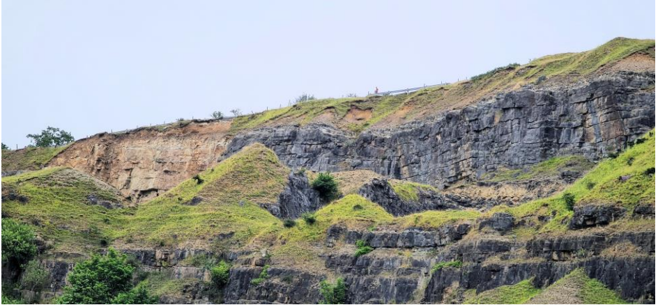
Figure 6. Large quarry near the end of the walk. A former road teeters above it
