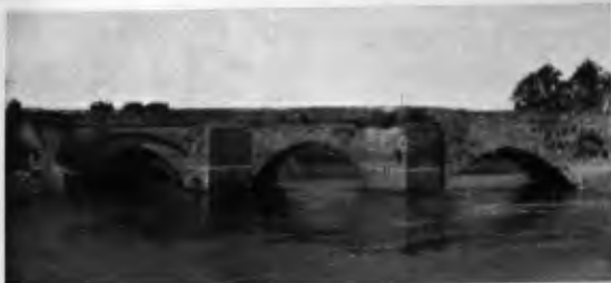
1. LUGG MILL BRIDGE. (Before restoration.)
