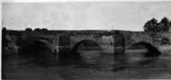
1. LUGG MILL BRIDGE. (Before restoration.)
