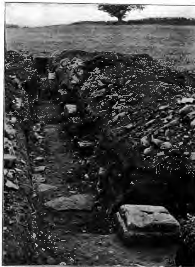
SITE 9. THE MOULDED BASE STONE AND N. AND S. DRAIN.
