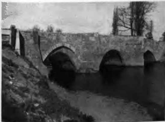
2. LUGG MILL BRIDGE. (After restoration.)
