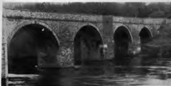
1. BREDWARDINE BRIDGE. (After restoration.)
