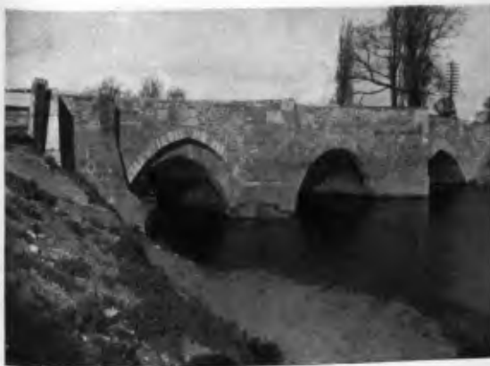
2. LUGG MILL BRIDGE. (After restoration.)
