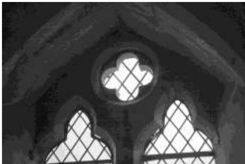
Figure 8 (left). The east window in the south wall of the chancel, showing the plate tracery that probably contained the Hugh de Breusa arms
