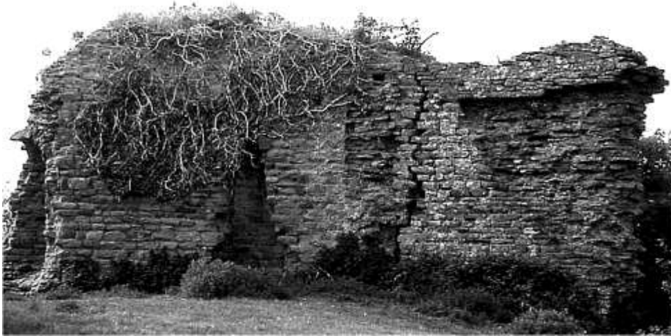
Figure 5. The interior of the north wall at Kilpeck Castle c.1982
