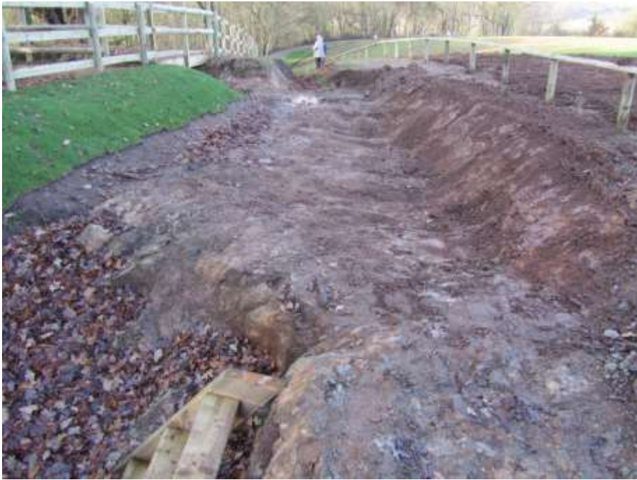
Plate 2.5 Wall of the disused Martley Pit in the main trench. Meta-igneous rocks of the Malverns Complex are exposed in the pit wall by the steps and in the rockhead pavement excavated above. View of the main trench looking north-west. (Moira Jenkins)
