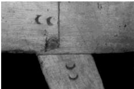
Figure 5 (left). Carpenters' marks in the larger barn
