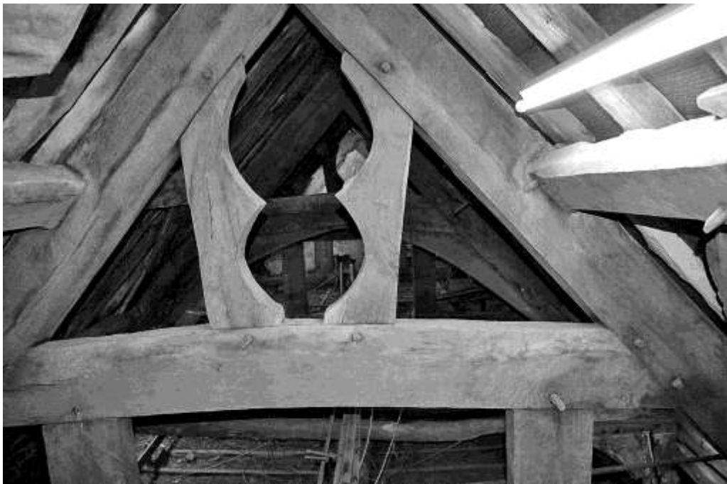
Figure 3. The Master's House, Ledbury. Dais truss looking east
