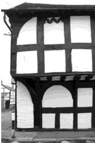
Figure 16. The Red Lion, Weobley. Side view of the crosswing showing the former trading hatch. This also shows how the jettied front has been under-built
