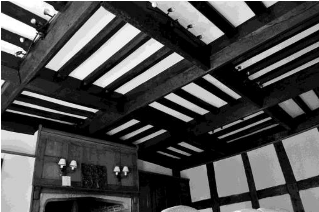
Figure 15. The Throne, Weobley. Counterchange ceiling in bay 7
