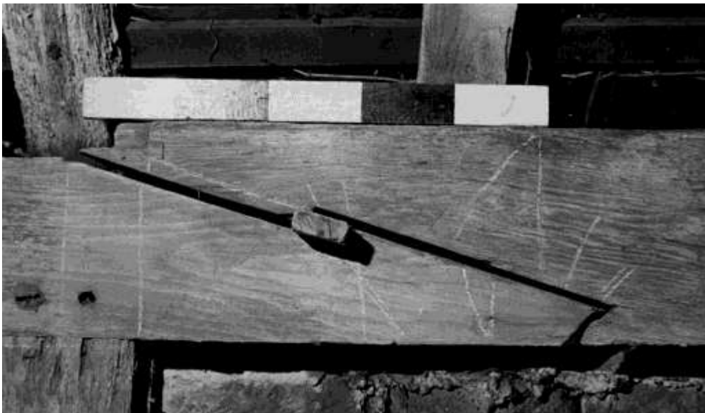
Figure 14. Detail of the arcade plate junction showing the splayed-and-tabled scarf joint
