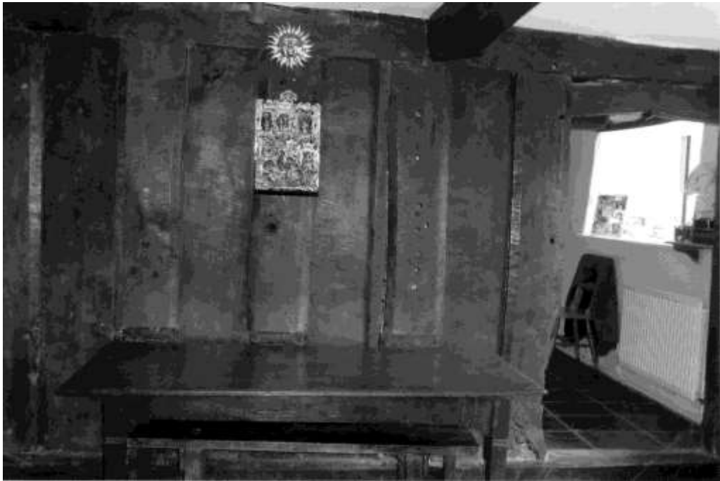
Figure 2. Plank and muntin screen and north doorway
