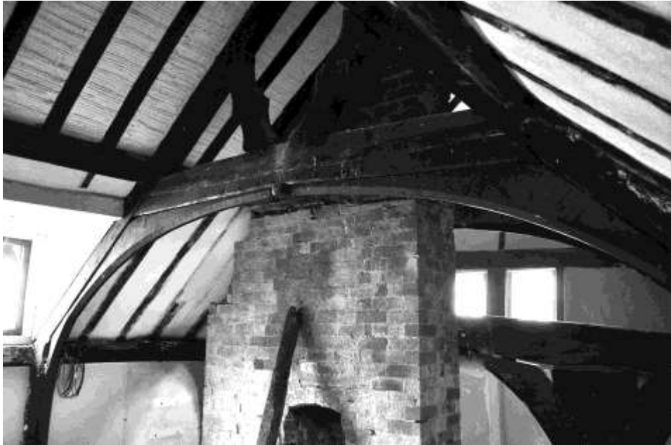
Figure 5. The principal truss over the hall in The Old Corner House. The upper part of the spere truss is visible behind the inserted chimney stack
