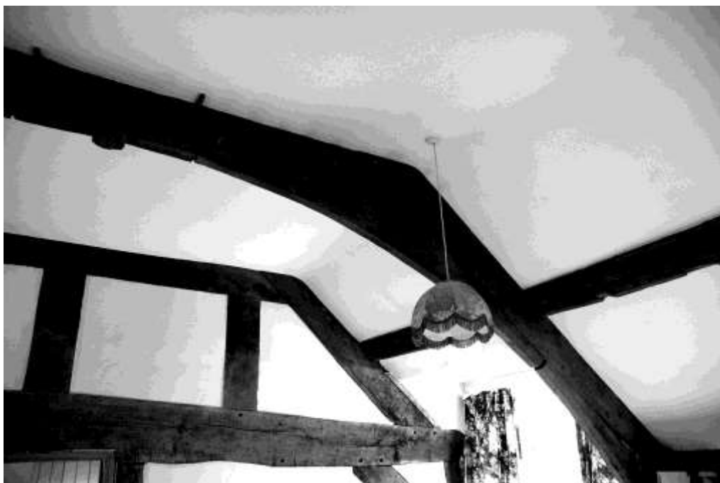
Figure 6. Double-arch bracing, with central boss, over the hall of Marlbrook House, Weobley
